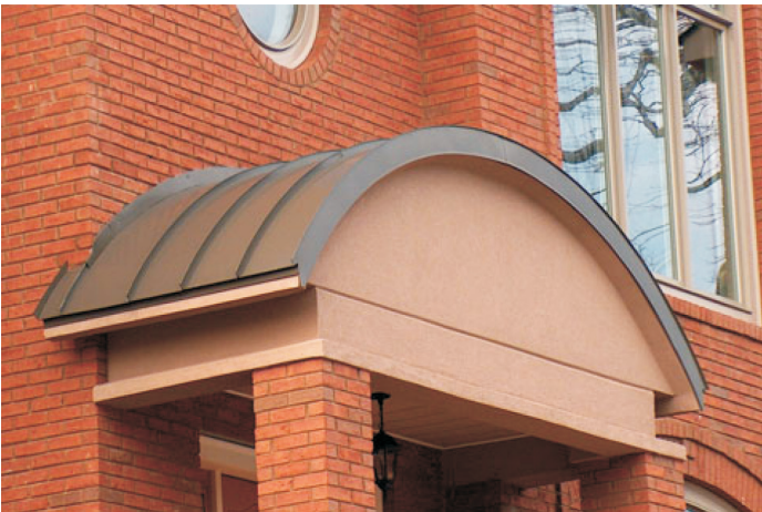
A typical barrel dormer on a private residence in the Atlanta area using our 1-1/2" mechanical seam US150 roof panel in 24ga galvalume steel. Note curved flashings.
