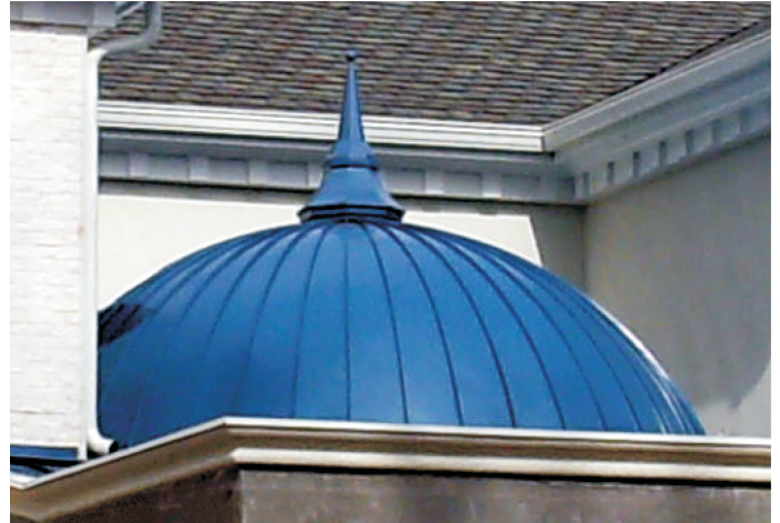
This dome project at a private residence in Atlanta, GA is fabricated from 24ga galvalume steel, standard paint color and using our 1" batten seam panels and caps.
